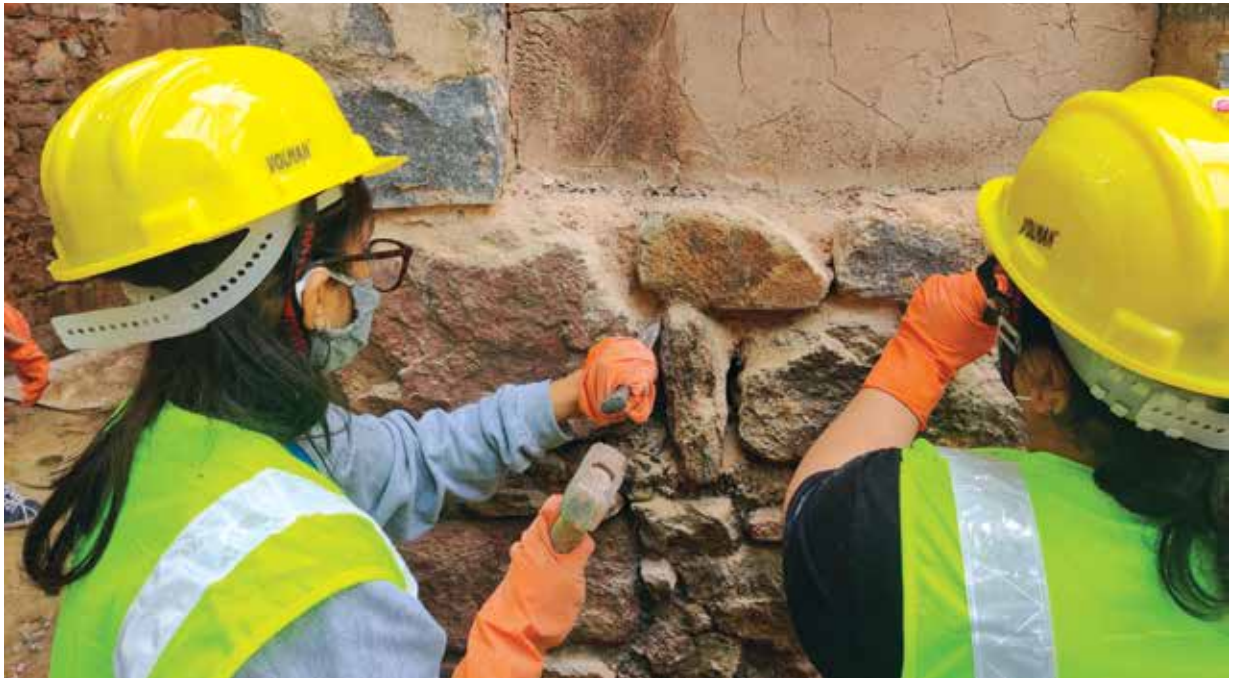
Students working on brick masonry on site
